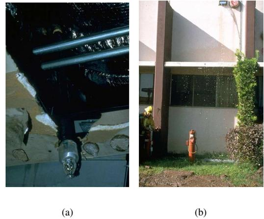
Figure 7. (a) Broken sprinkler in Olive View hospital after Northridge earthquake in 1994 (Courtesy National Information Service for Earthquake Engineering (NISEE), University of California, Berkeley). (b) Sprinkler pipe leakage after an aftershock of the 1994 Northridge earthquake near Olive View Hospital (Courtesy NISEE, University of California, Berkeley).
