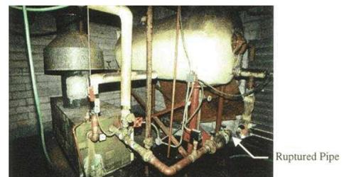
Figure 8. Ruptured pipe of the supply line to a 3000 liter storage tank in the roof top of mechanical room – 2001 Nisqually earthquake [23].
